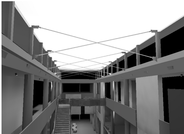
Raised Roof and Exposed Crossing Bracing System
