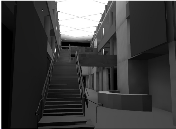
View from Staircase
